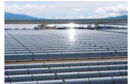
Spanish sun farm: In Granada Province, parabolic mirrors supply up to 200,000 people with solar power.
