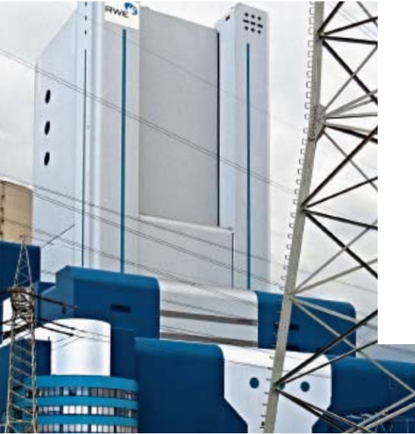
CO 2 scrubbing: A CO 2 capture pilot plant should start operating in 2009 at RWE Power's Niederaussem lignite power plant.
