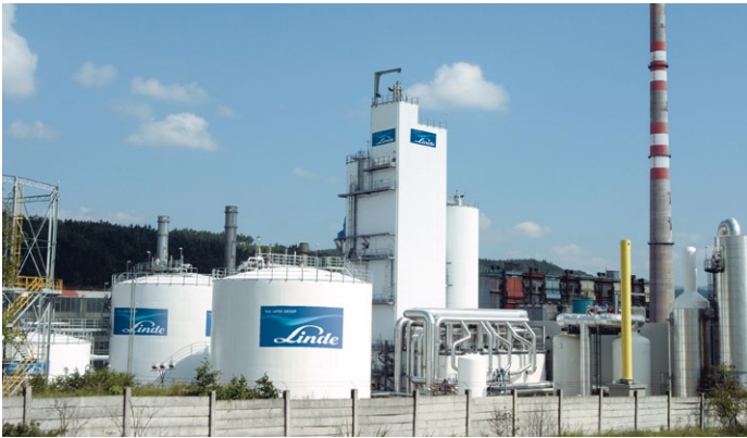
Figure 7: A cryogenic air separation plant
