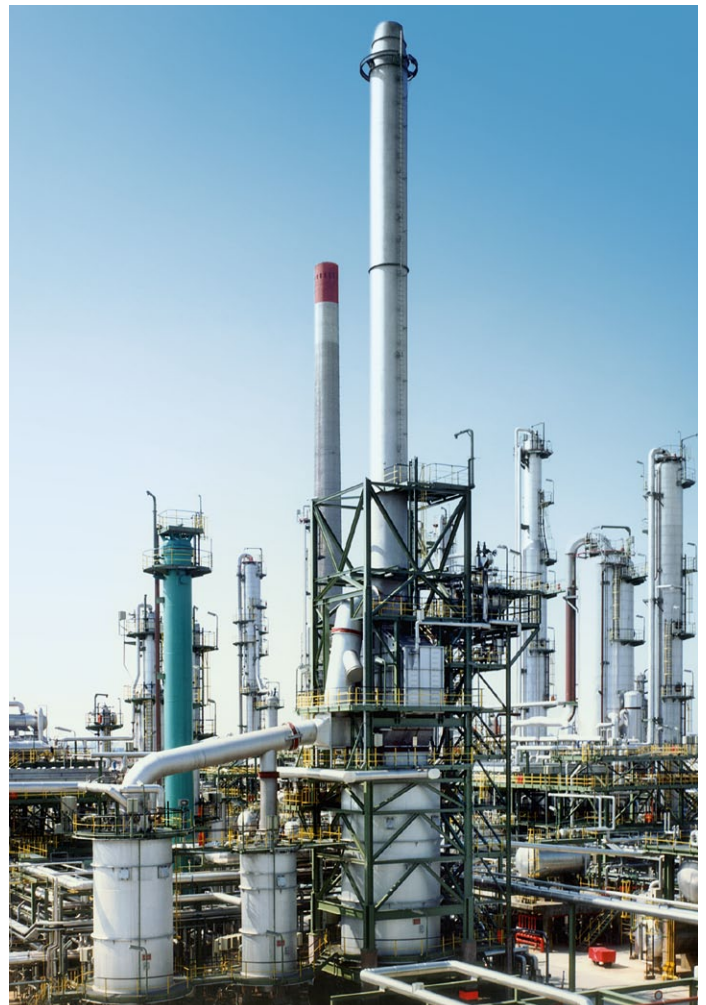
Figure 37: Refinery with oxygen enrichment for FCC
