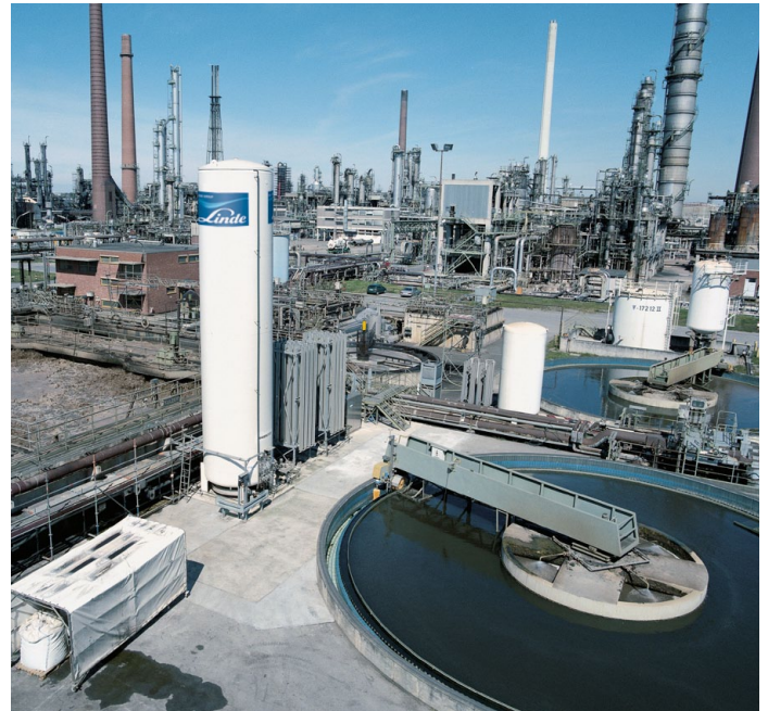
Figure 42: Using pure oxygen for intermittent denitrification in the wastewater treatment plant of a refinery
