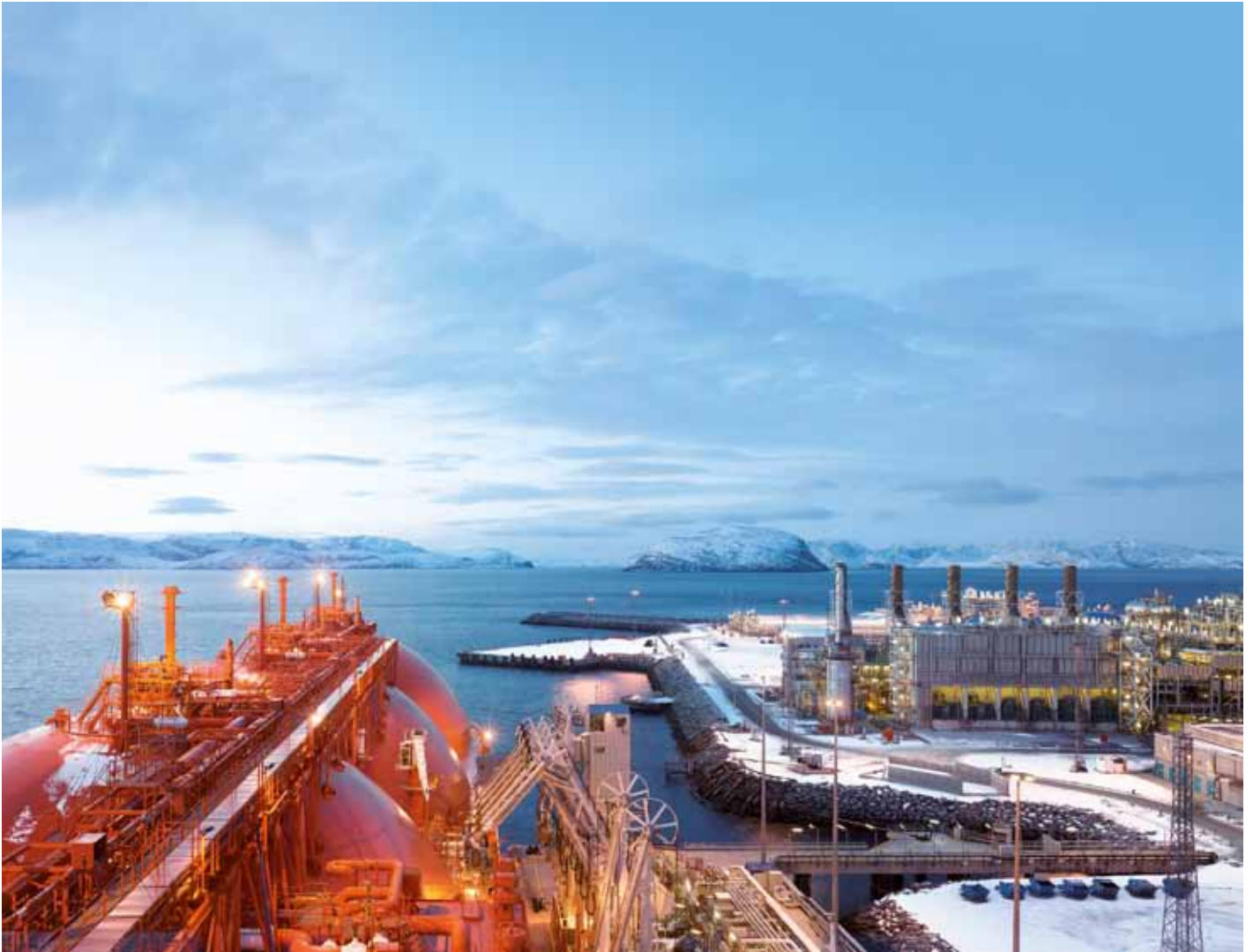
A global journey that starts in Norway: Cryogenically frozen LNG from Hammerfest travels the globe in the spherical tanks of the Arctic Princess (top left). 12,000 cubic metres of natural gas are pumped into the carrier's hold each hour. The LNG is stored in massive storage tanks (opposite).
