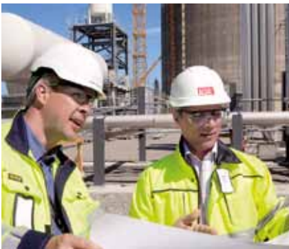
Everything under control: Engineers from Linde's Swedish company AGA Gas AB at the construction site of the Baltic Sea's first LNG terminal.
