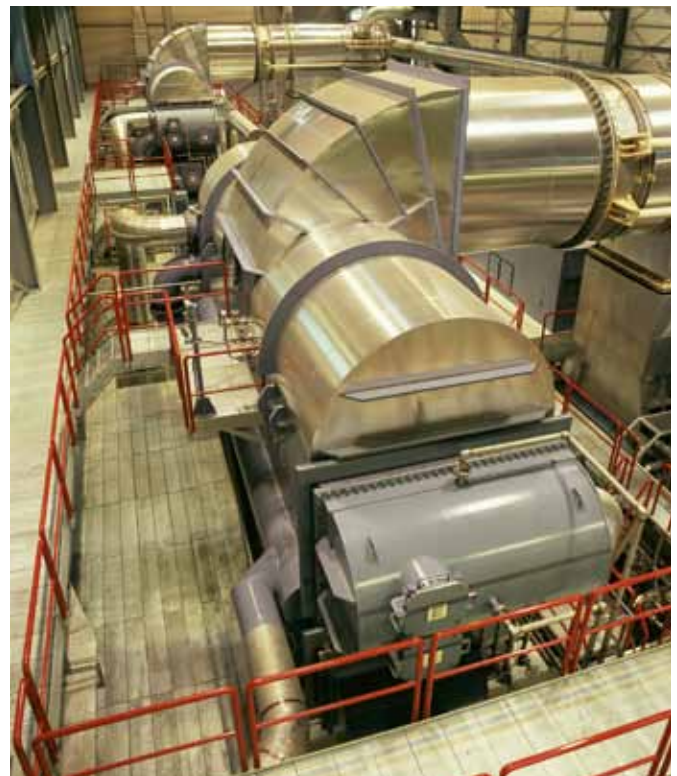
Harnessing the Earth's heat: Linde supplies air coolers, heat exchangers, pipelines and electronic controls for the Kirchweidach geothermal power plant in southern Germany (above). Cryostar is responsible for installing the turbines and generators (below).
