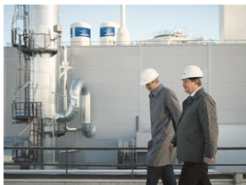
Linde constructed a new air separation unit on the grounds of Russian steel manufacturer NLMK.
