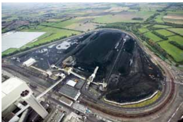
Feedstock: The Drax coal-fired power plant in the UK (above) is considered one of the most efficient worldwide. There are plans to construct an innovative oxyfuel plant with CO 2 separation (right) in North Yorkshire, England. On completion, it will be one of the world's most important CCS demo projects.
