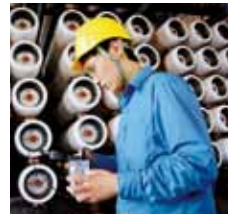
Water on standby: A technician checks the reverse osmosis equipment required for seawater desalination (top). Before the raw water (left) can be used, it must pass through Linde's CO 2 enrichment system, SOLVOCARB® (right, front).
