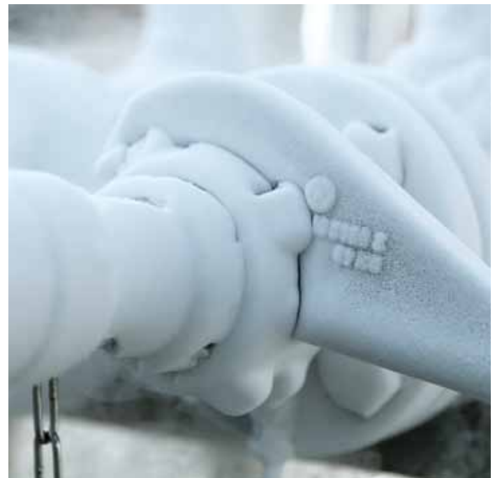
Temperature extremes: The liquid nitrogen in the tankers is maintained at minus 196 degrees Celsius (left). Damp air condenses to form frost on the ice-cold pipes in August 2011 (bottom). Following delivery (top), the cryogenic cargo is vaporised for the inerting step. Heat exchangers warm the N 2 up to 40 degrees Celsius.
