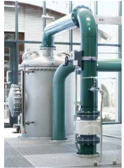
Water on standby: A technician checks the reverse osmosis equipment required for seawater desalination (top). Before the raw water (left) can be used, it must pass through Linde's CO 2 enrichment system, SOLVOCARB® (right, front).
