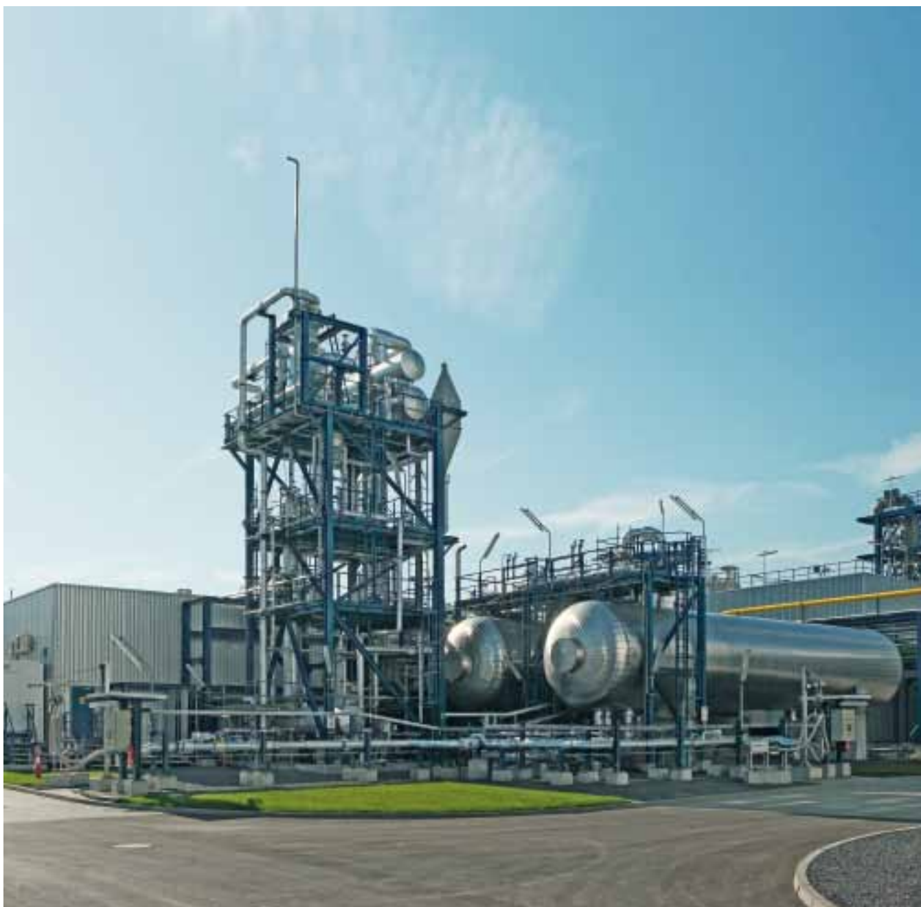
↳ Coal power with reduced CO 2 emissions – oxyfuel pilot project in Schwarze Pumpe, Germany.
