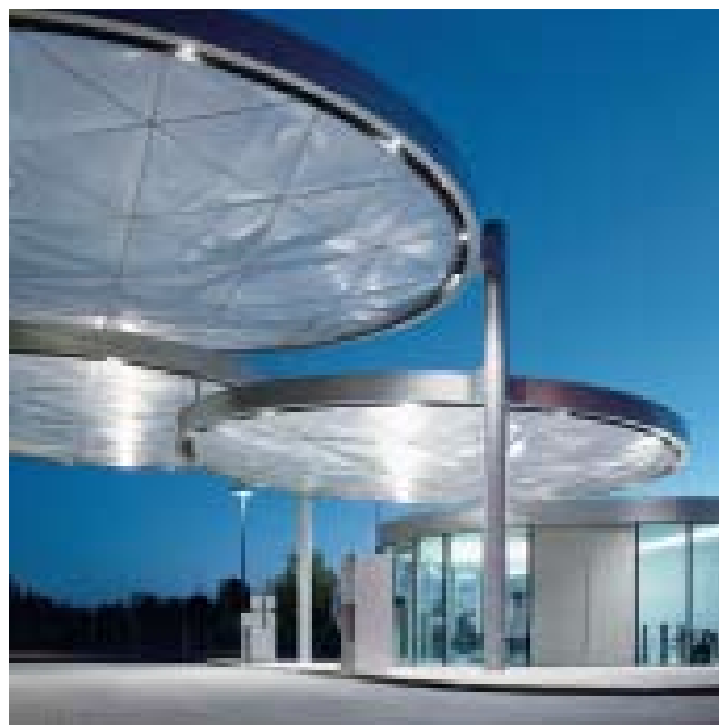
↳ The Linde Hydrogen Center in Unterschleißheim near Munich puts new hydrogen refuelling solutions through the paces.
